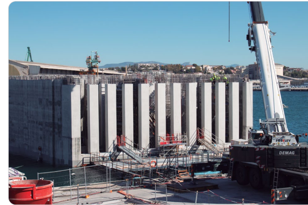
Pictures courtesy of Bouygues
