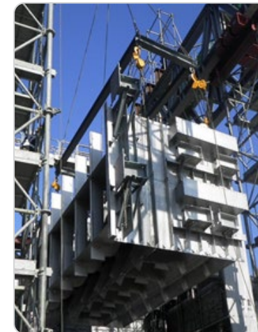
Water intake of a dam. Picture courtesy of NSSC.
