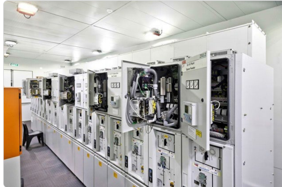
Picture courtesy of the Southern Africa Stainless Steel Development Association
